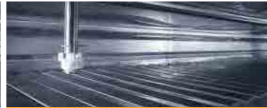
Clean-in-Place (CIP) Upgrade for Existing Freezers
