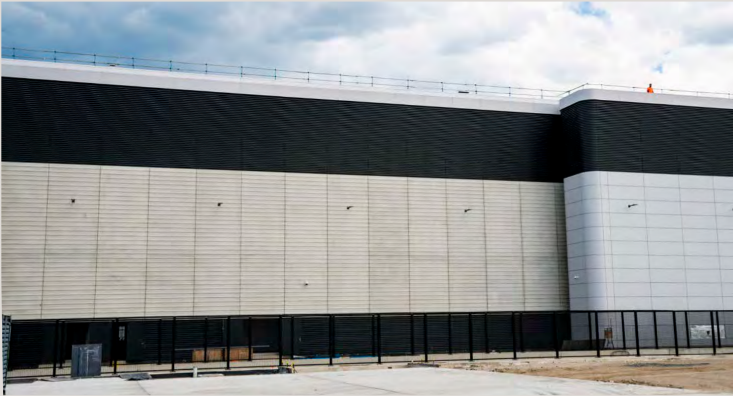
Western Sydney Airport Transport Infrastructure | NSW
