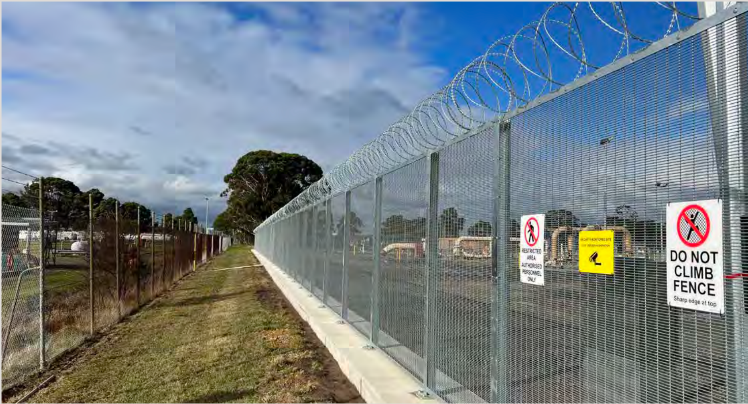
APA Dandenong South Utilities | VIC
