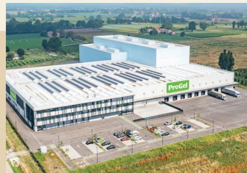
Automated Logistics Centre: Arceto di Scandiano (IT)
