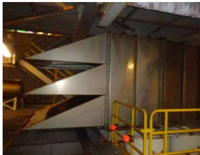
Intake Filter House of GT2: Due to the location between decks, the feasibility of increasing the size of the air intake filtration system was limited.
